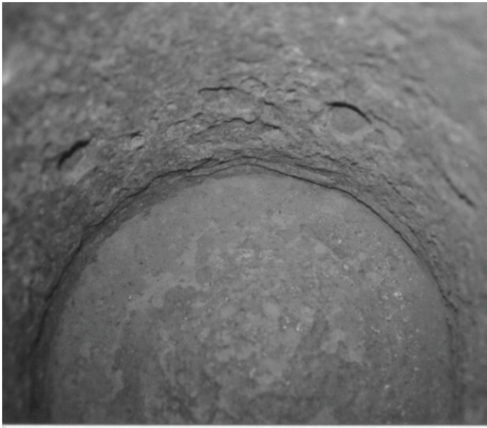
Figure 16: Corrosion at the bottom of a condemned carbon dioxide cylinder
